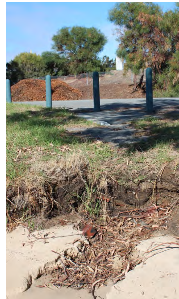
IMAGE 16. STORMWATER RUN OFF, BALBUK WAY
